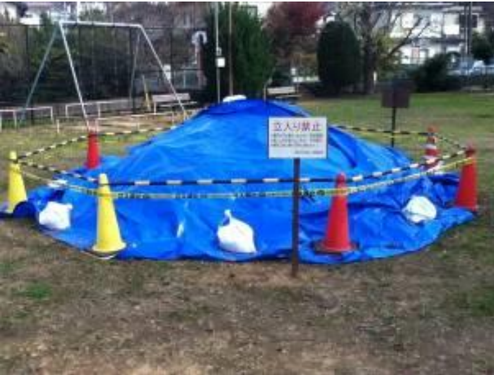
Contaminated soils covered by blue-colored sheet in Children's park, 0.49uSv/h , Chiba-Pref.
