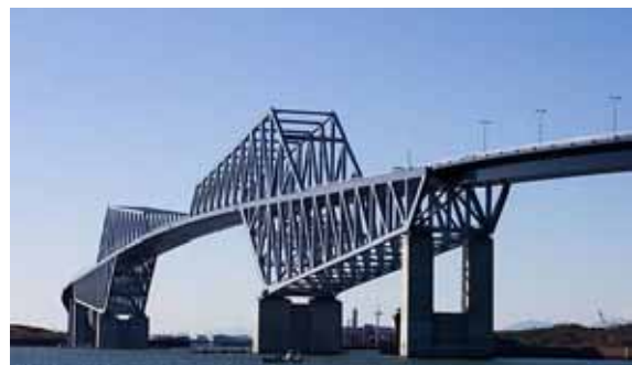
Tokyo Gate Bridge
